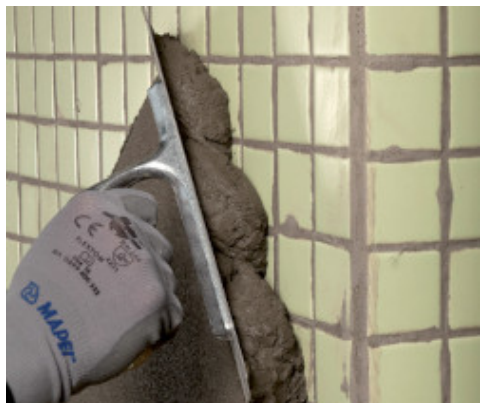
Applying Planitop 200 on glass mosaic
