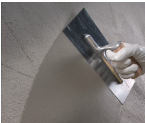
Applying Planitop 200 on concrete
